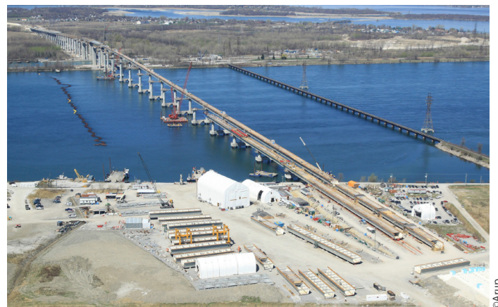
Staging yard used to facilitate preparation for launching of the box girders.
