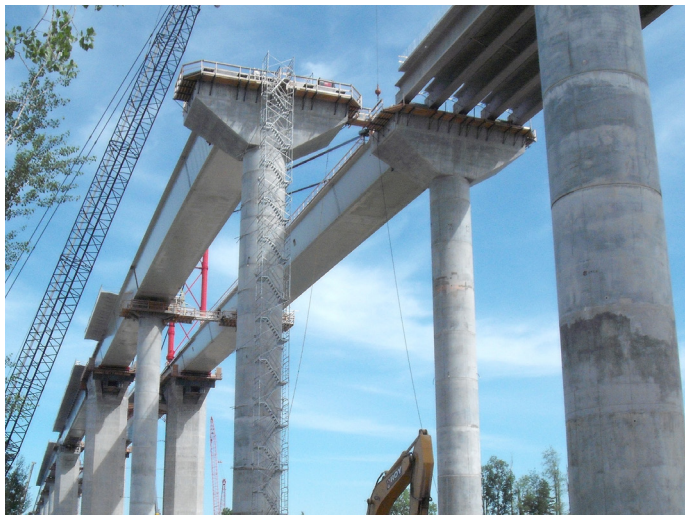
Top: Completed Beauharnois Canal Bridge looking westward | Bottom Left: Post-tensioned piers providing nearly 40 metres of clearance over the Beauharnois Canal Bottom Right: Work continues on the Beauharnois Canal Bridge through the night, to meet project milestones
