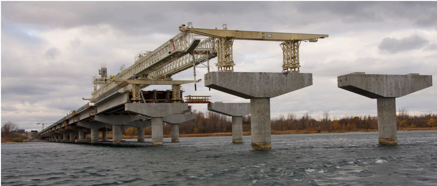
Installation of NEBT beams over the St. Lawrence River using a launching gantry
