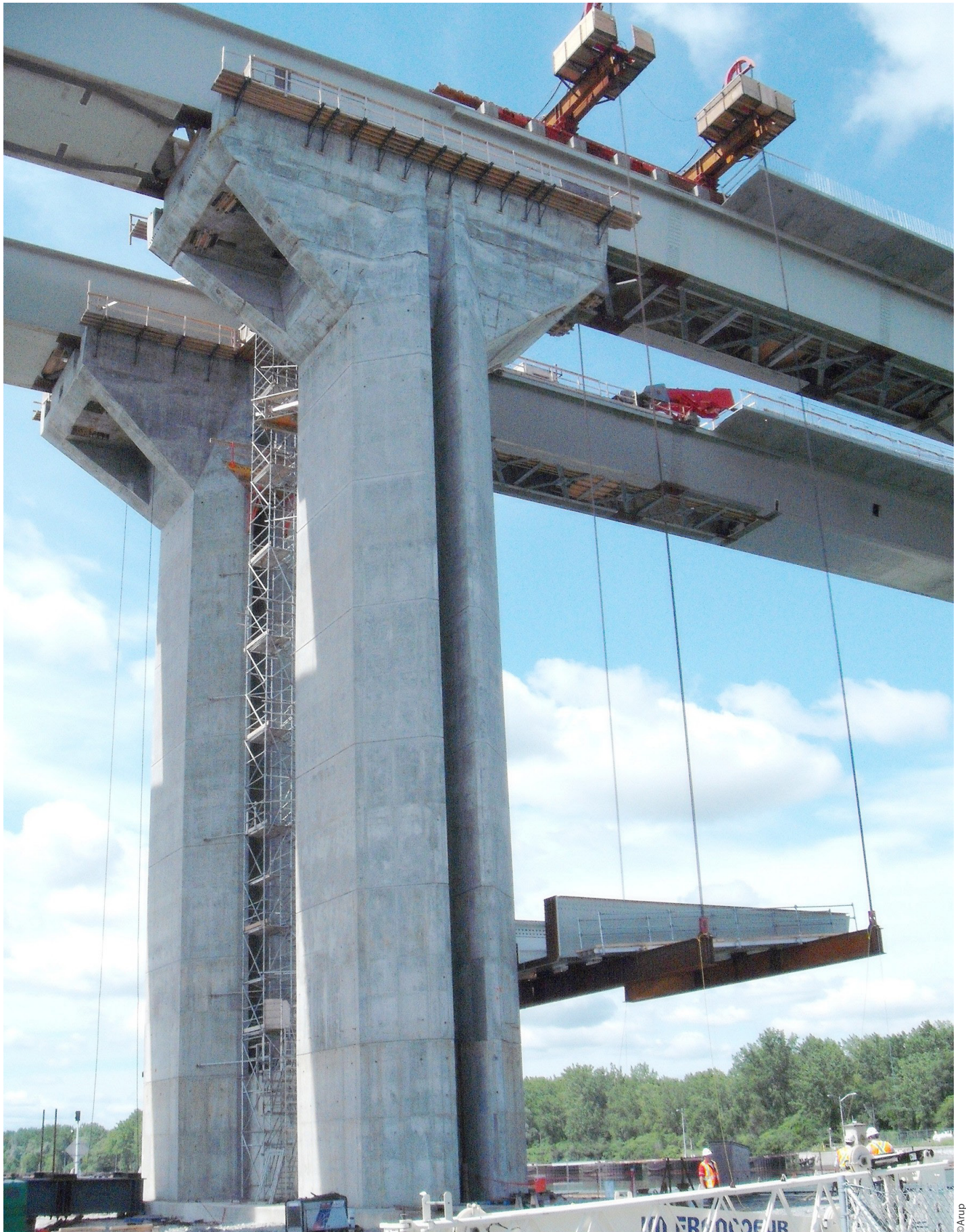
Lifting of steel haunch section at one of the monolithic main piers for Beauharnois Canal Bridge
